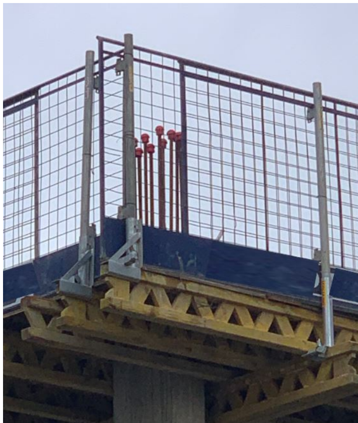
Figure 1. An example of cross-contamination of edge protection systems.
